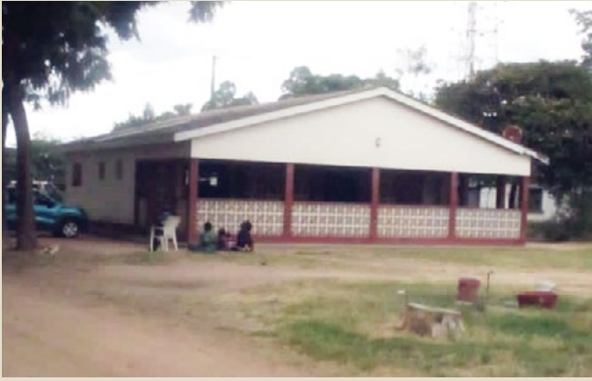
Mahusekwa Circuit Court building
