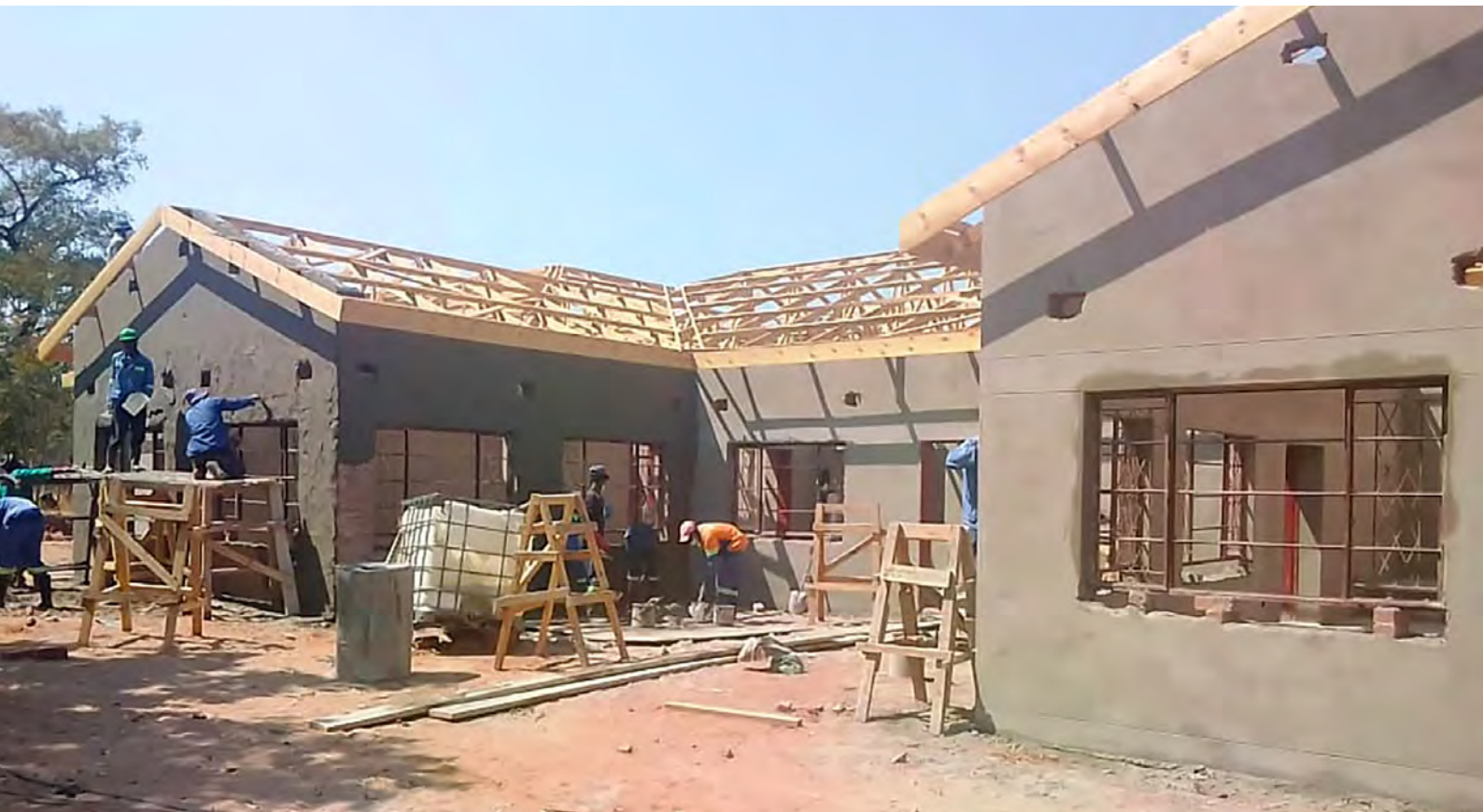
Lupane Court house under construction
